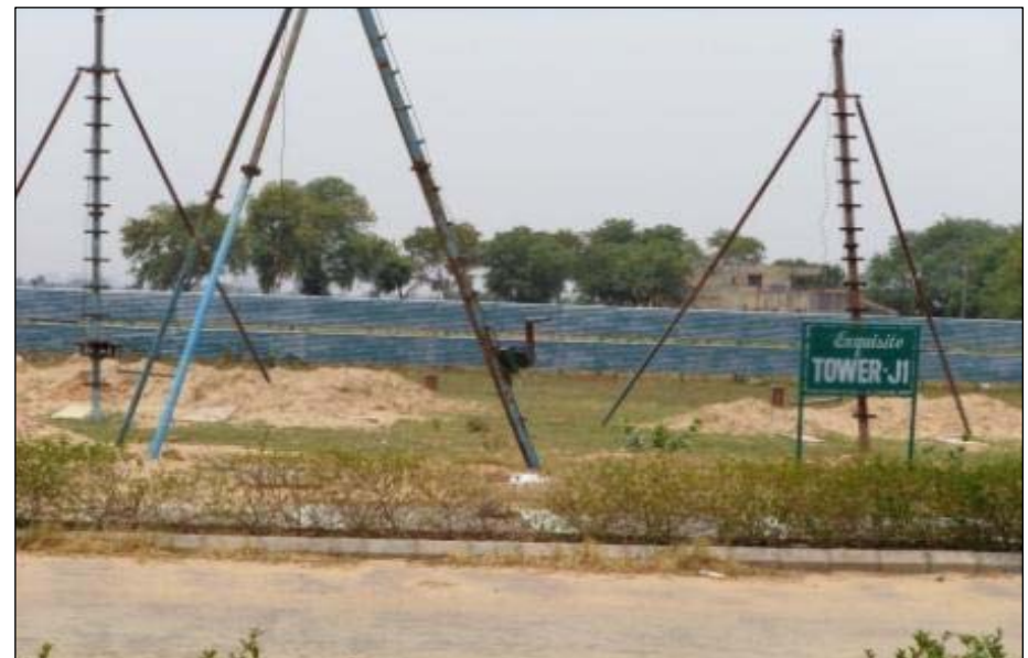
EXQUISITE, NC-2, GURGAON – Piling in progress
