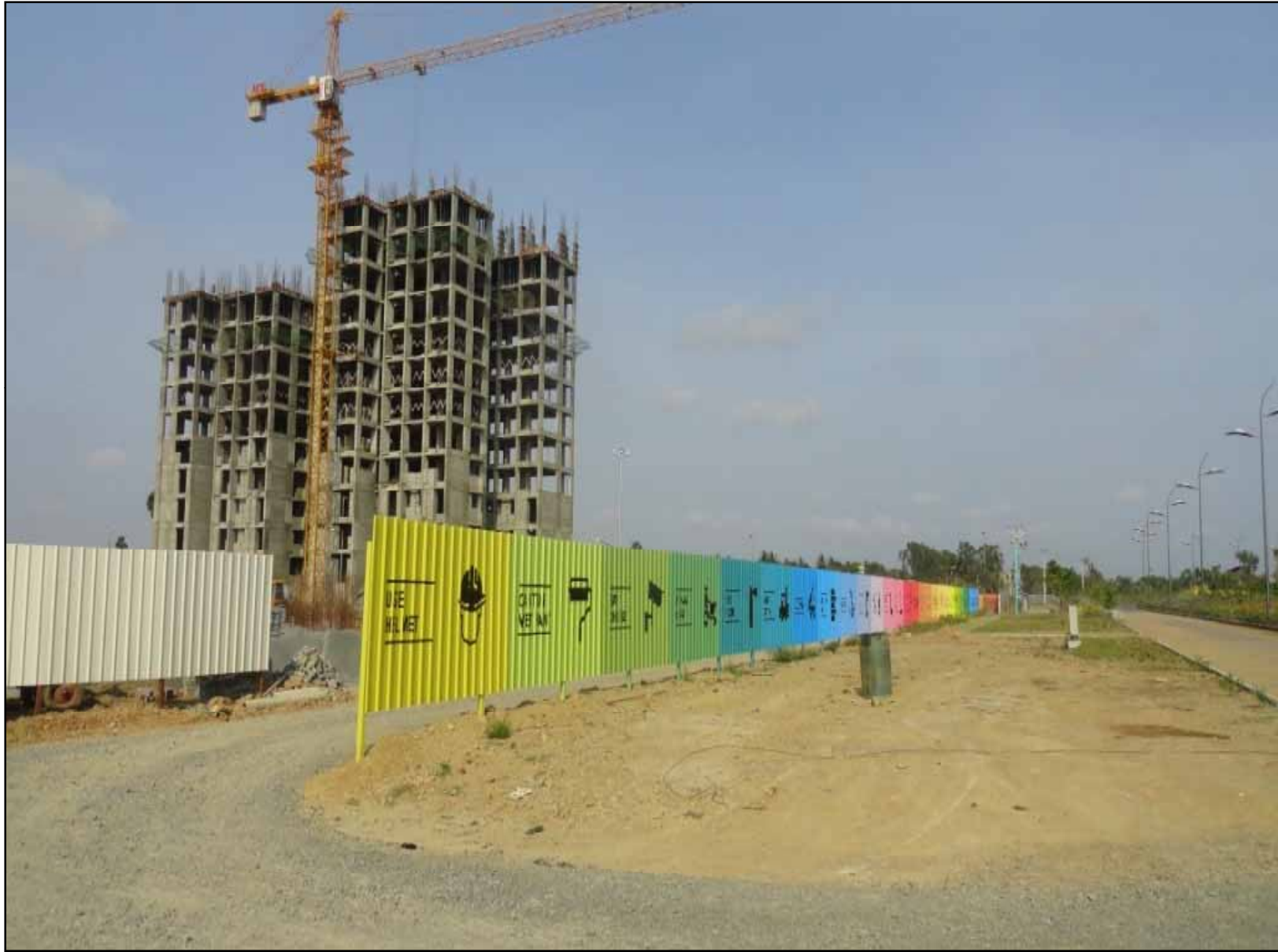
UW GARDENS, CHENNAI – Structure work in progress
