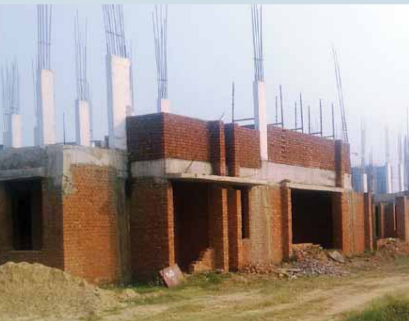
Structure work in progress in the rows of 500 sq. yd. villas
