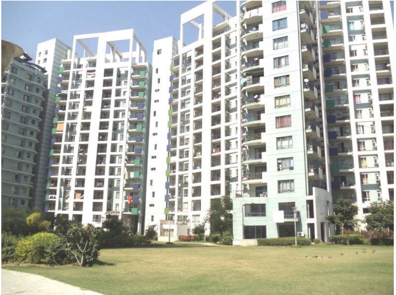
View from project entrance - Tower 5, 6, 7 in background
