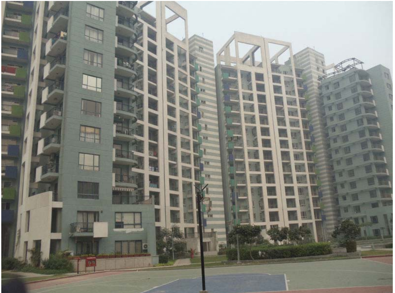
Tower 9, 10, 11 - Tower 10, 11 advance stage of completion
