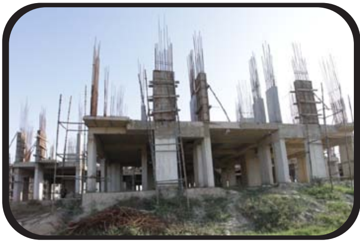
◀ Tower B1 1st floor column casting work in progress
