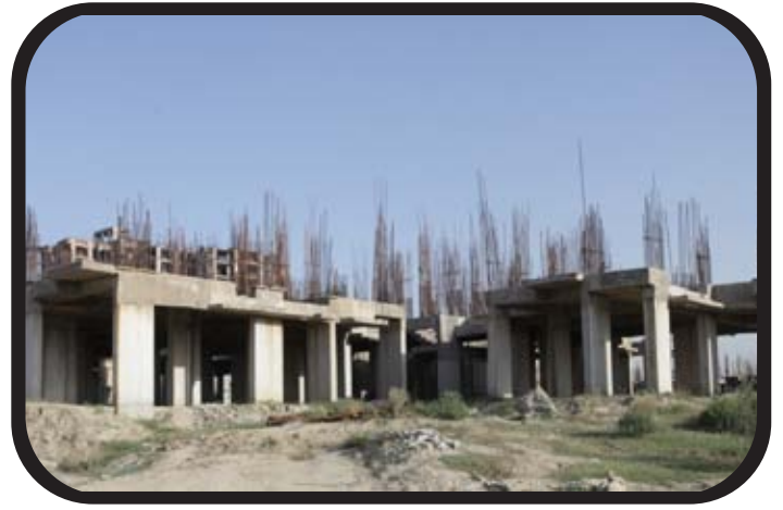
Tower B2 Ground floor slab casting completed ▶
