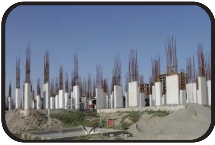
◀ Tower B3 Ground floor column casting in progress
