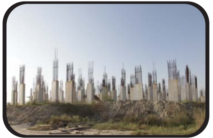
Tower C Ground floor column casting in progress. ▶
