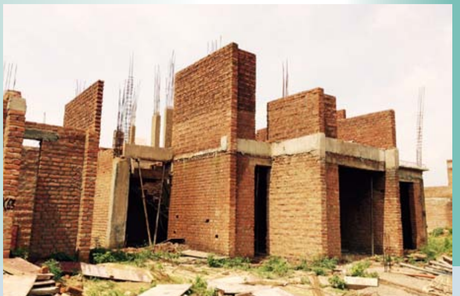
Masonry work in progress.
