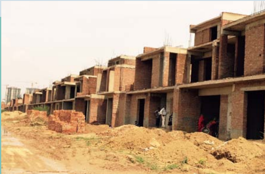
Structure work at various stages in different villas.
