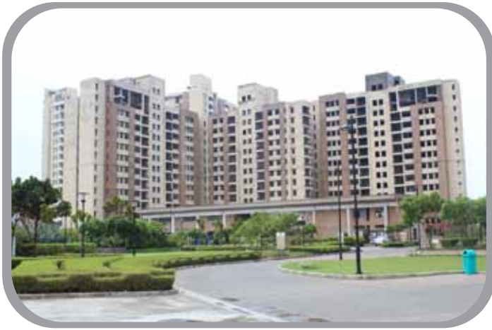
project periphery road
