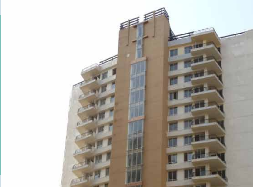
Tower 5 External view of the Tower
