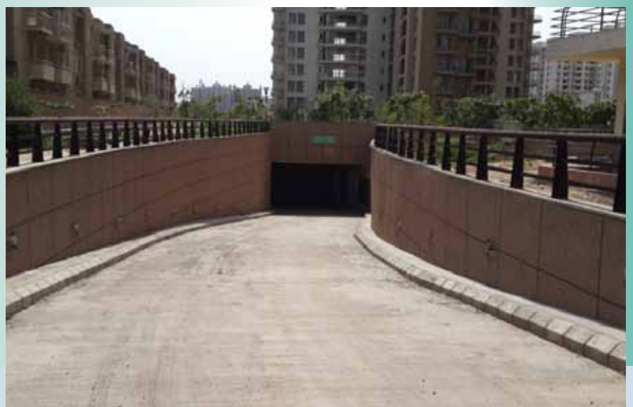
Basement Ramp View of the entry ramp for Towers 4 - 8
