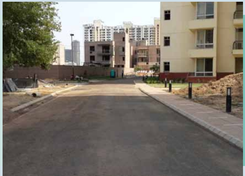
Internal Road View of the road towards Tower 8
