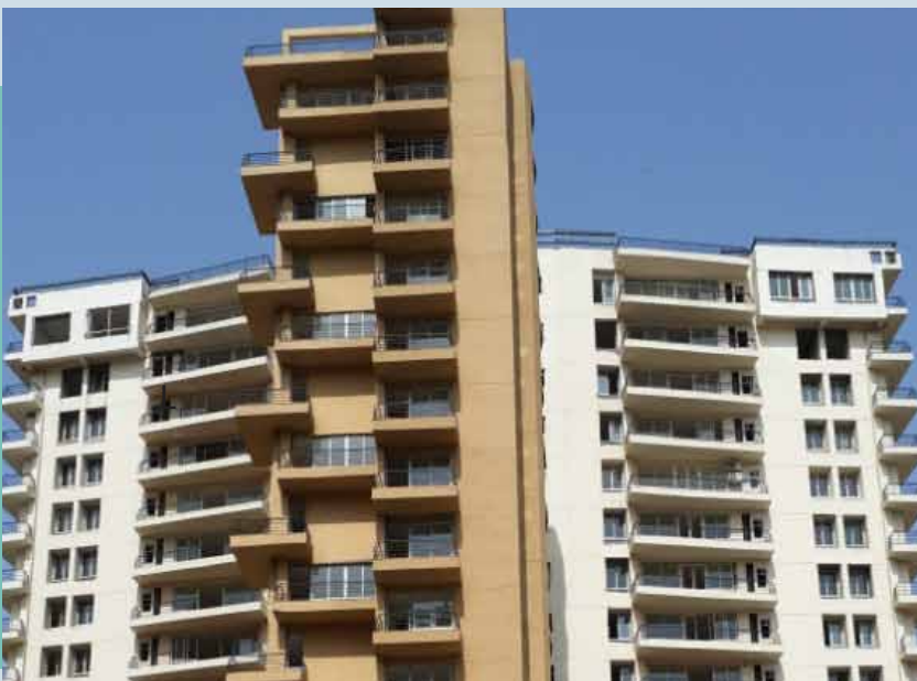
Tower 8 External view of the Tower
