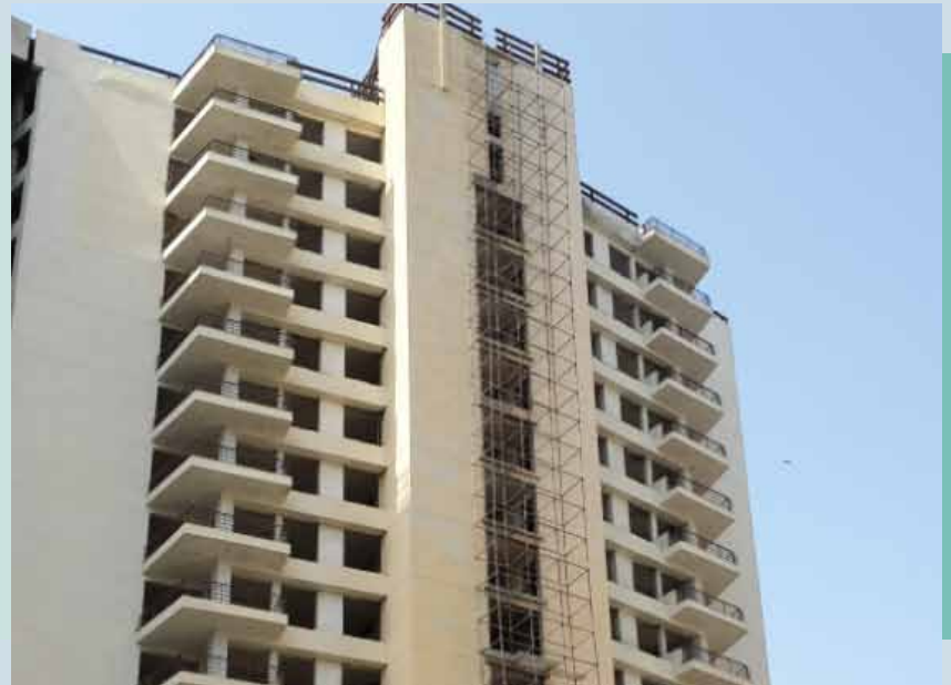
Tower 7 External view of the Tower
