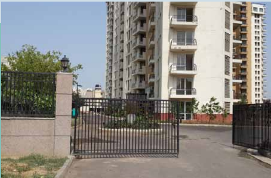
Entrance Gate-Towers 4 - 8 View of the entrance gate
