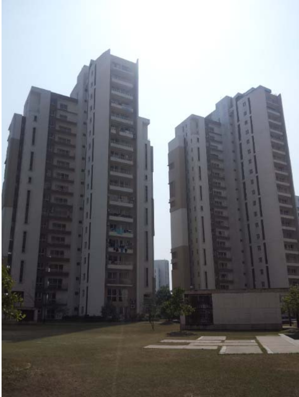
Horizons Tower 1 & 2(back side)
