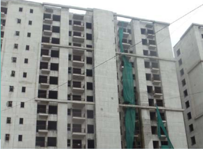
A-6 Structure, external plaster completed. Aluminum frames work in progress.
