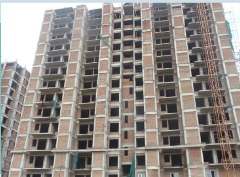
C-2 Brickwork and internal plaster in progress.
