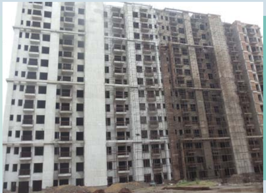
B1,B2 External plaster work in progress.
