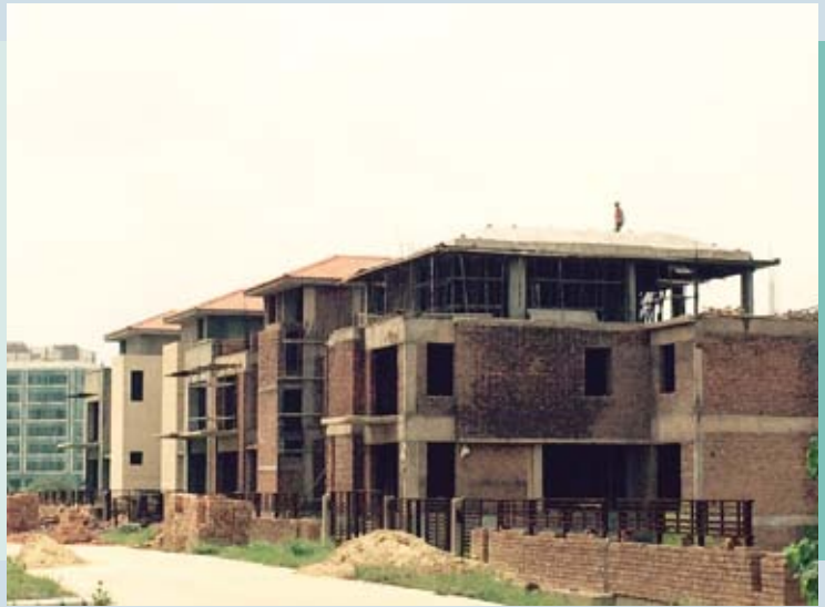
Roof slab casting in progress.
