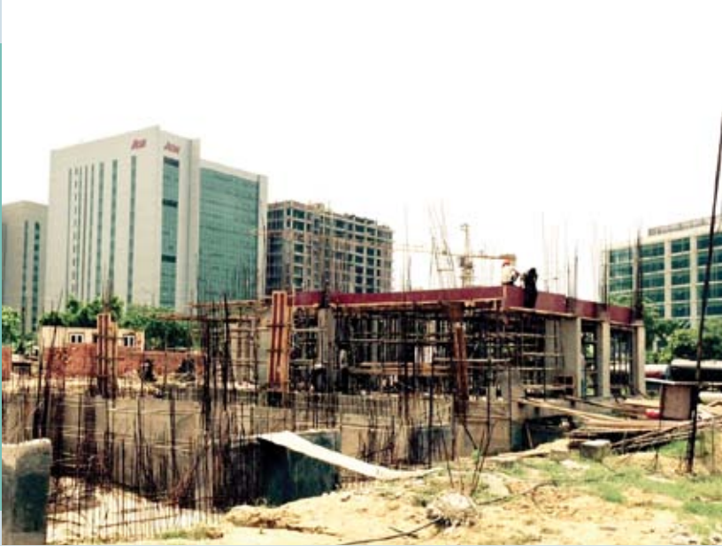
Roof slab shuttering & reinforcement work in progress.
