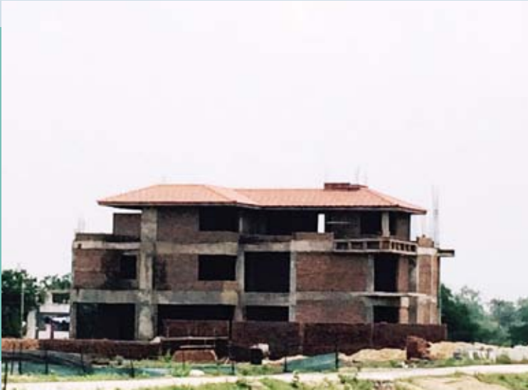
Masonry work in progress in the Villas.
