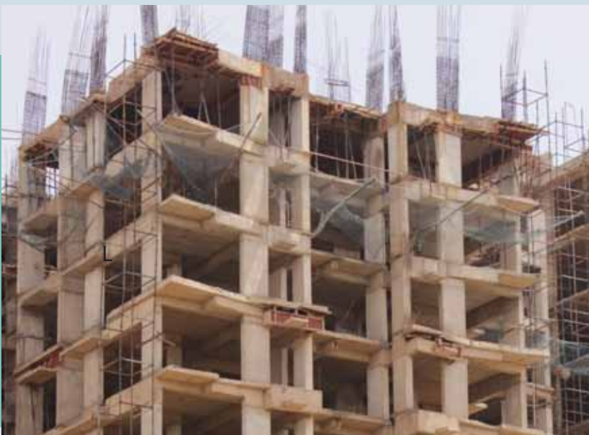
Tower A5 Civil structure is in progress.
