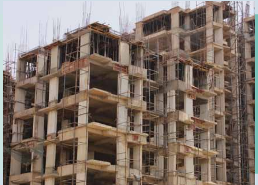
Tower A4 6th floor roof in progress
