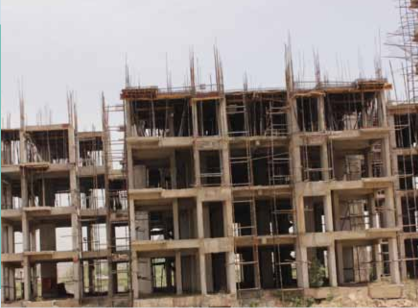
Tower A3 3rd floor roof in progress
