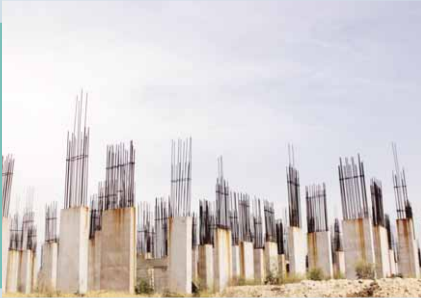
C Block Foundation work completed.
