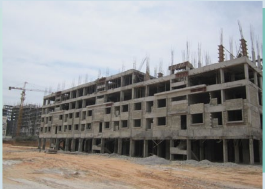
Structure and brick work in progress for Tower 1 to 3
