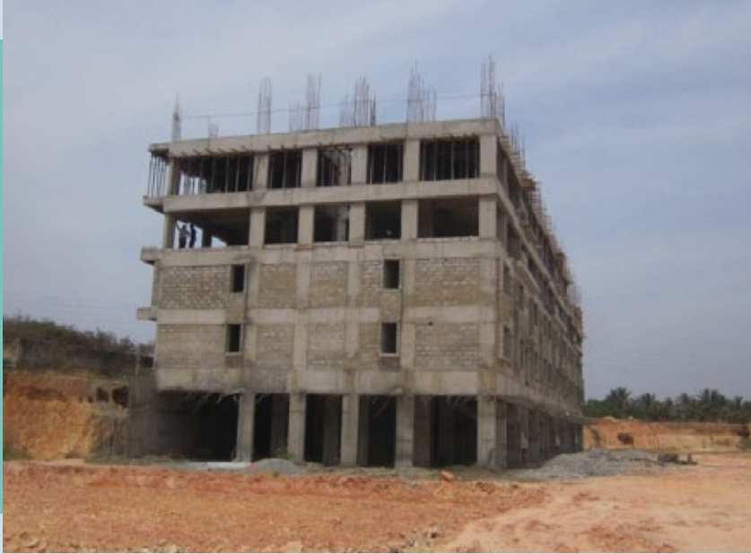
Structure and brick work in progress for Tower 1 to 3
