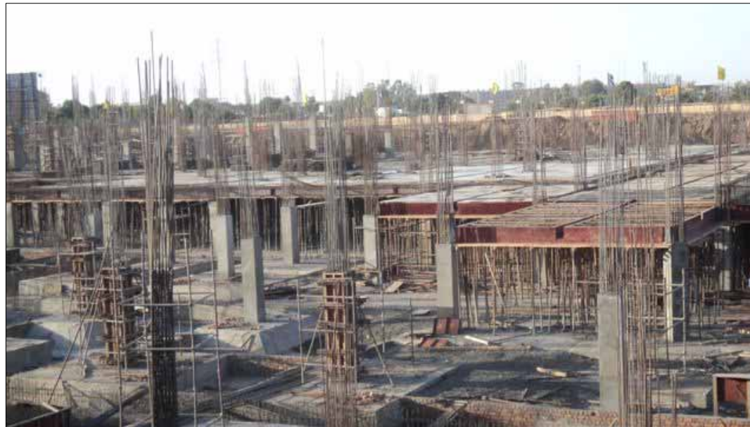
GIP, Bhopal – Piling / Structure in progress
