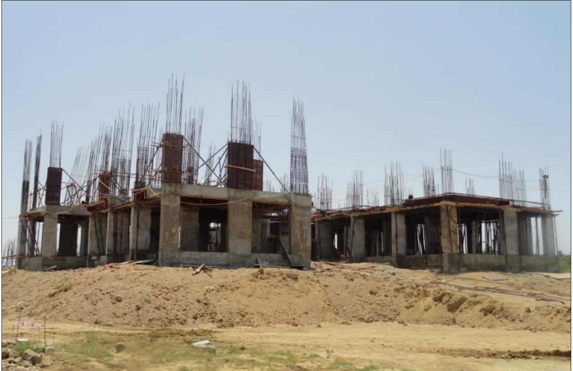
UW GARDENS, CHENNAI – Structure work in progress
