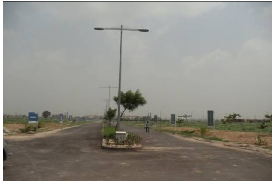
ASPEN GREENS, MOHALI – Development work in progress
