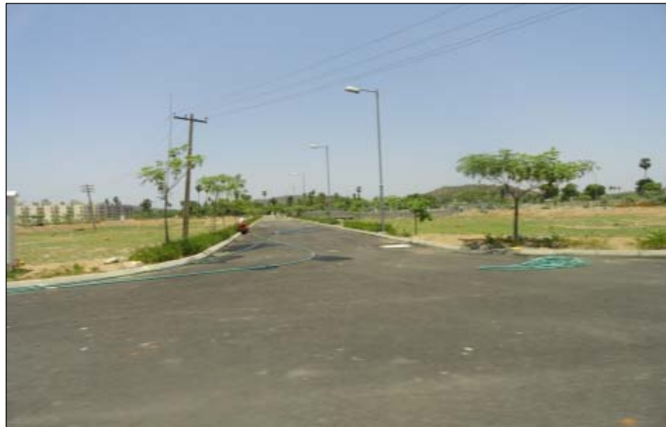
ASPEN GREENS, CHENNAI – Handover in progress
