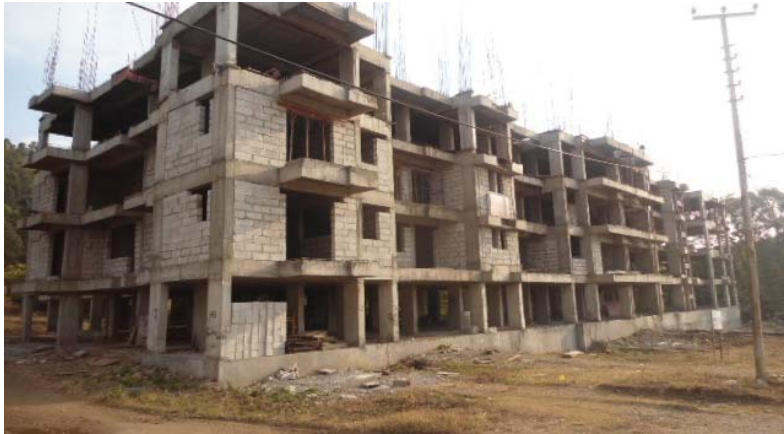
Residences Dehradun Structure work in progress
