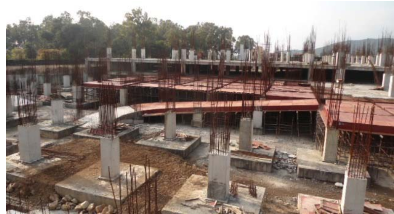
GIP Dehradun Structure work in progress
