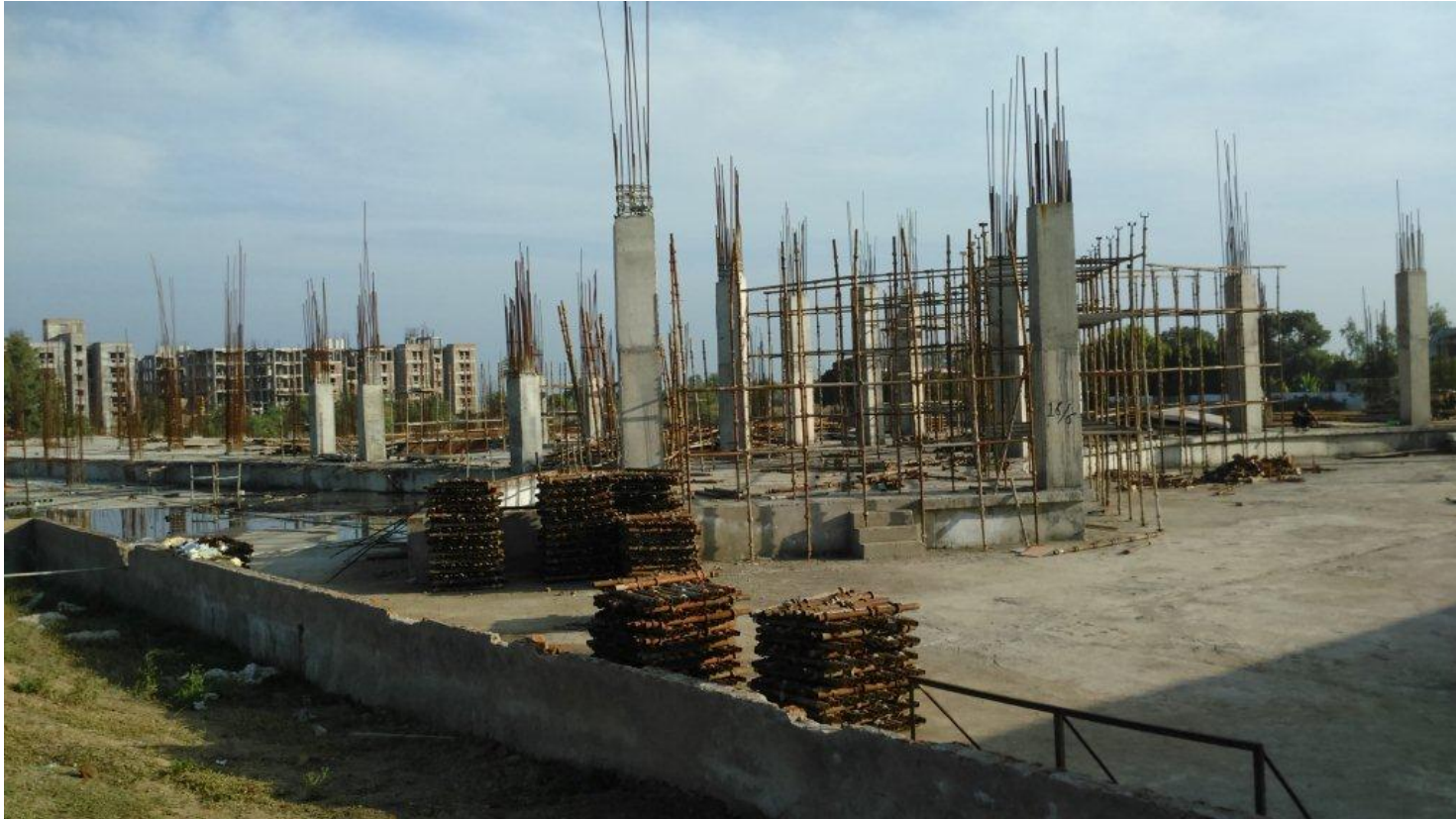
GIP – Piling/ Structure work in progress
